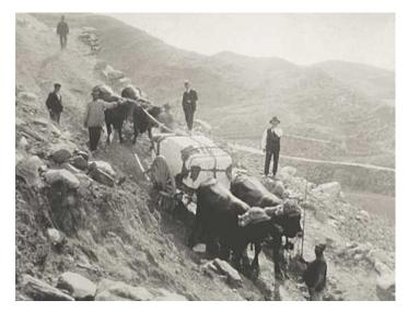
from the town of Fines to the quarries through the dangerous Rambla del Castillo. The marble company carried out works to widen and reinforce the road so that carts and carts could circulate through them to transport the marble from quarries five kilometers from the factory.
